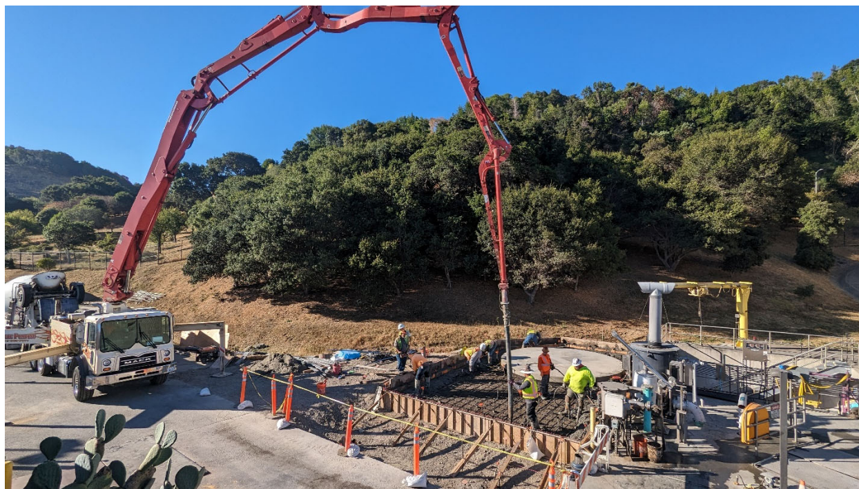
Liquid organic waste concrete pour for new above-grade storage tank.
