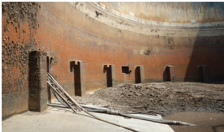
Digester No. 2, Final Stages of Initial Cleaning
