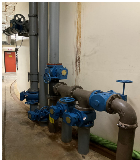
Digester No. 2 Process Piping Valve Replacements
