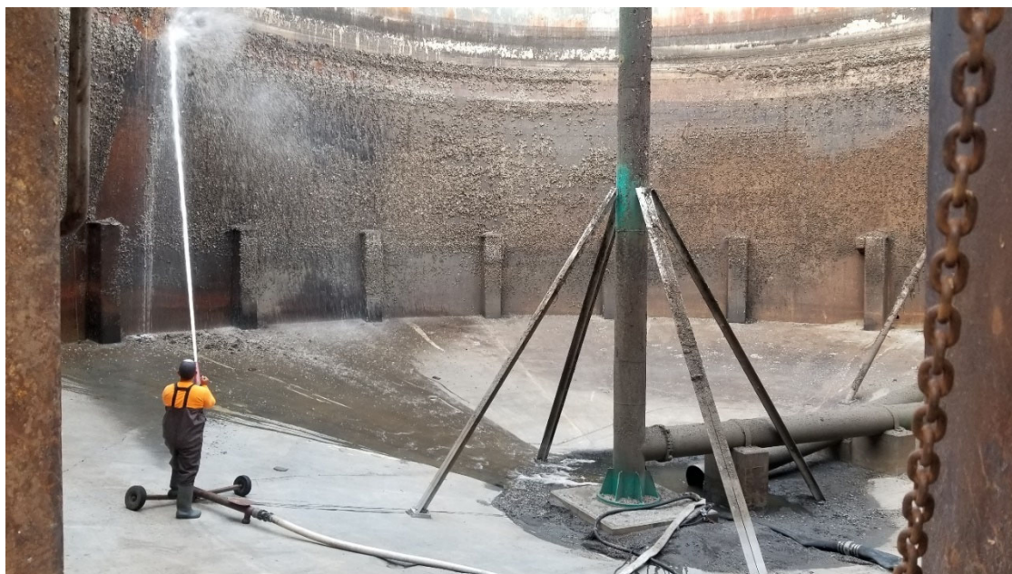
Inside Digester No. 2, cleaning of wall deposits
