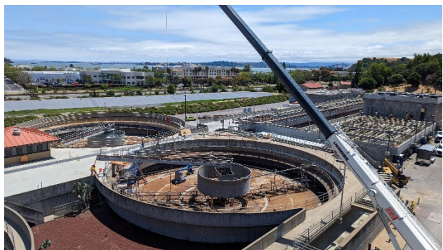
Removal of Walkway Bridge in Secondary Clarifier No. 2
