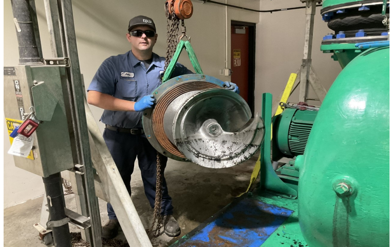
Digester No. 2 Mixing Pump Refurbishment
